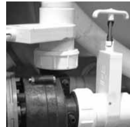
Slice Valve and Pump Union
