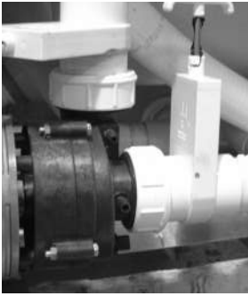
Slice Valve and Pump Union
