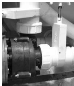
Slice Valve and Pump Union
