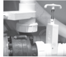
Slice Valve and Pump Union
