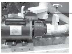
To relieve an airlock situation, loosen the pump union on the discharge of the pump. This pump union is indicated by an arrow in the picture. Water should leak out of the union once the air has been removed. Tighten the union and test the pump for proper operation. Repeat this process if needed.
