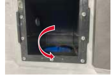
Turn Filter Counter-clockwise to Remove
