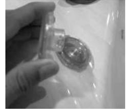
3. Either the whole Laminar Flow Jet Assembly pops out: Rinse it out and inspect it. Or, if only the outer ring comes off: Remove internal Jet insert with a pair of needle nose pliers and inspect it.
