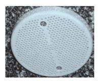
With the power to the spa off, remove the two screws holding the screen in place. Soak the screen in white vinegar and rinse thoroughly with water
