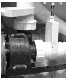
Slice Valve and Pump Union
