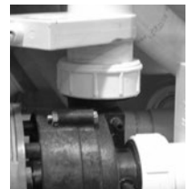
Slice Valve and Pump Union
