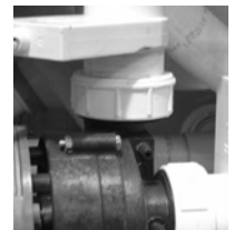
Slice Valve and Pump Union
