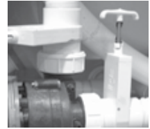
Slice Valve and Pump Union
