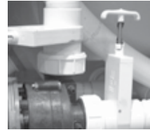
Slice Valve and Pump Union
