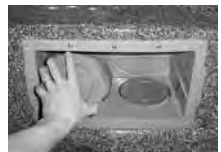
Install Eco Pur filter on left side.
